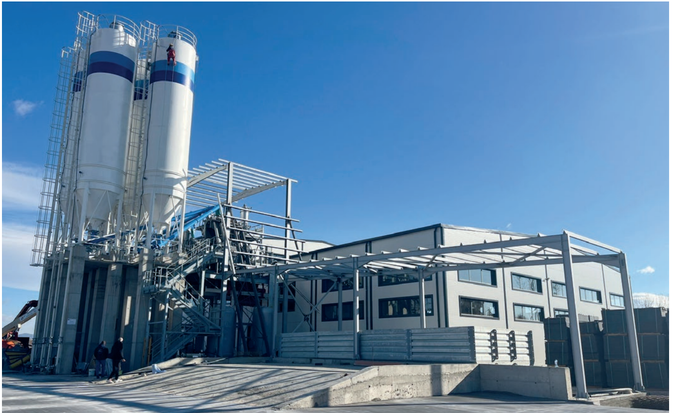
View of the new concrete block production facility in Zhitnitsa
