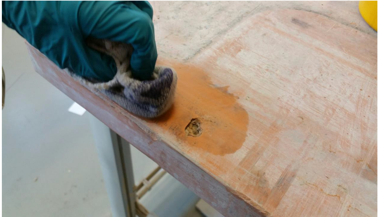
Step 2: Clean the surface near the damaged area
