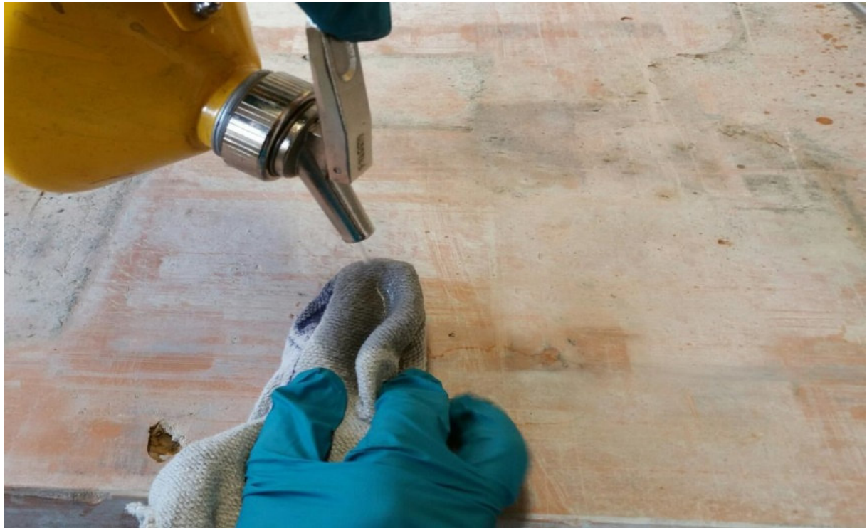
Step 1: Soak a cloth with acetone
