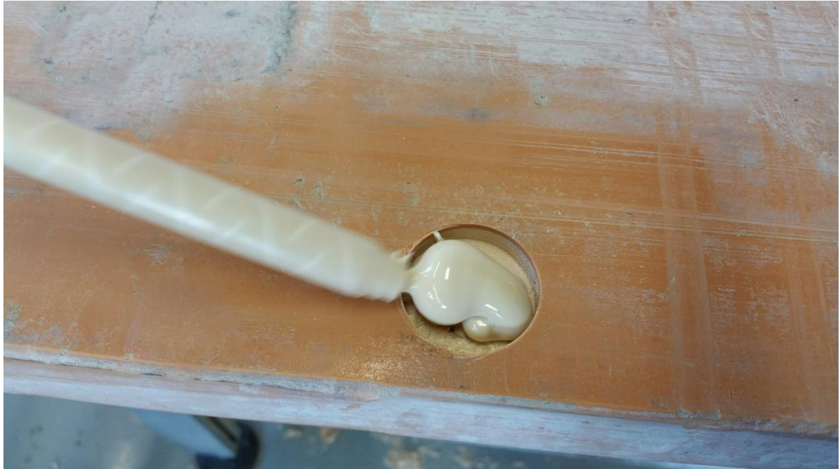
Step 6: Fill the drillhole with the repair material
