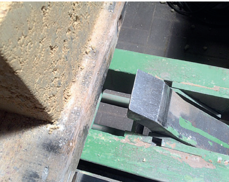
Steel pawls frequently develop a sharp edge on the top side over the course of time.
