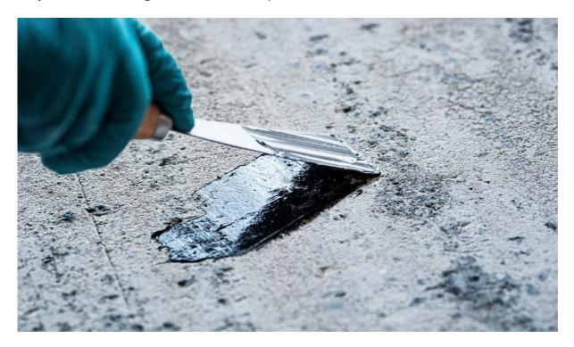
Step 4: Use a spatula to cleanly remove the excess material and smooth out the area
