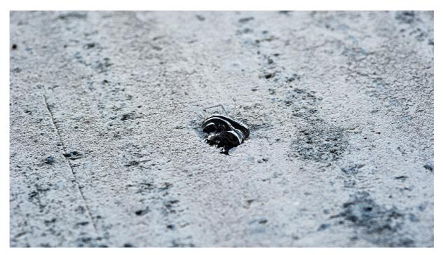
**Step 3:** Fill the damaged area with the repair material
