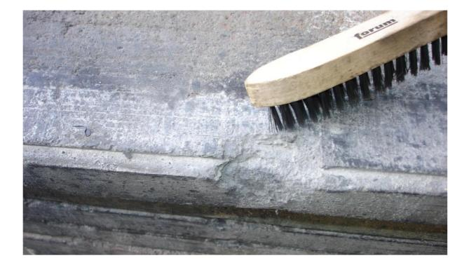
Step 1: Clean the surface near the damaged area
